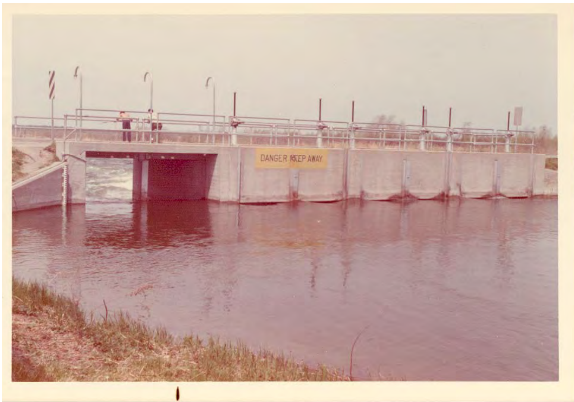
Red Lake Dam (May 1972)
