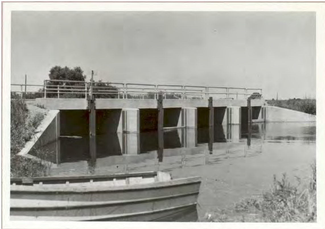
Upstream view of Red Lake Control Structure (July 1941)
