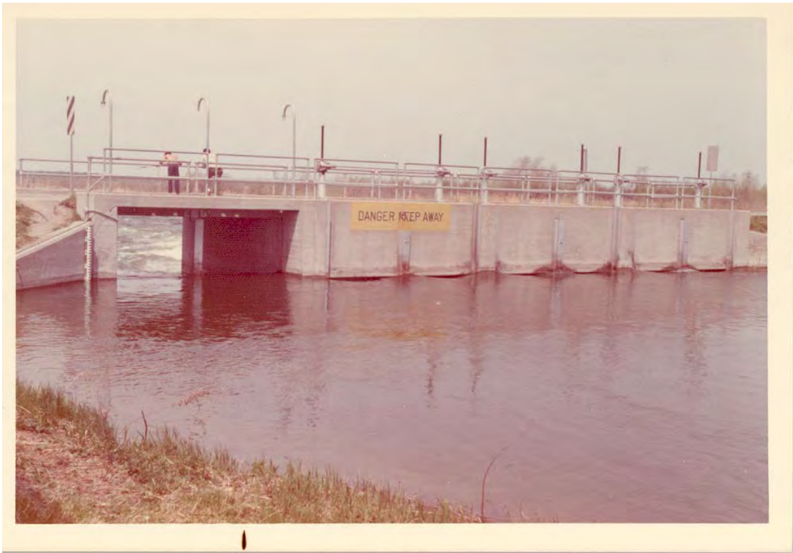
Red Lake Dam (May 1972)
