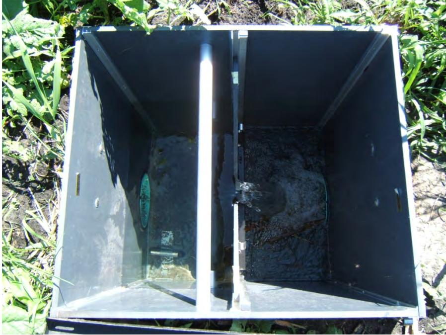
**Figure 12. Bachand Tile Drainage Water Control Structure**
