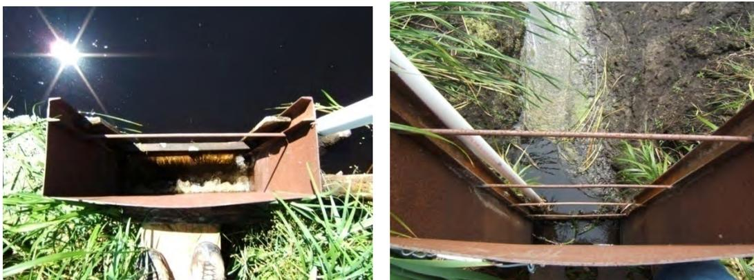
**Figure 29. Surface Drained Wild Rice Paddy Outlet Structure**
