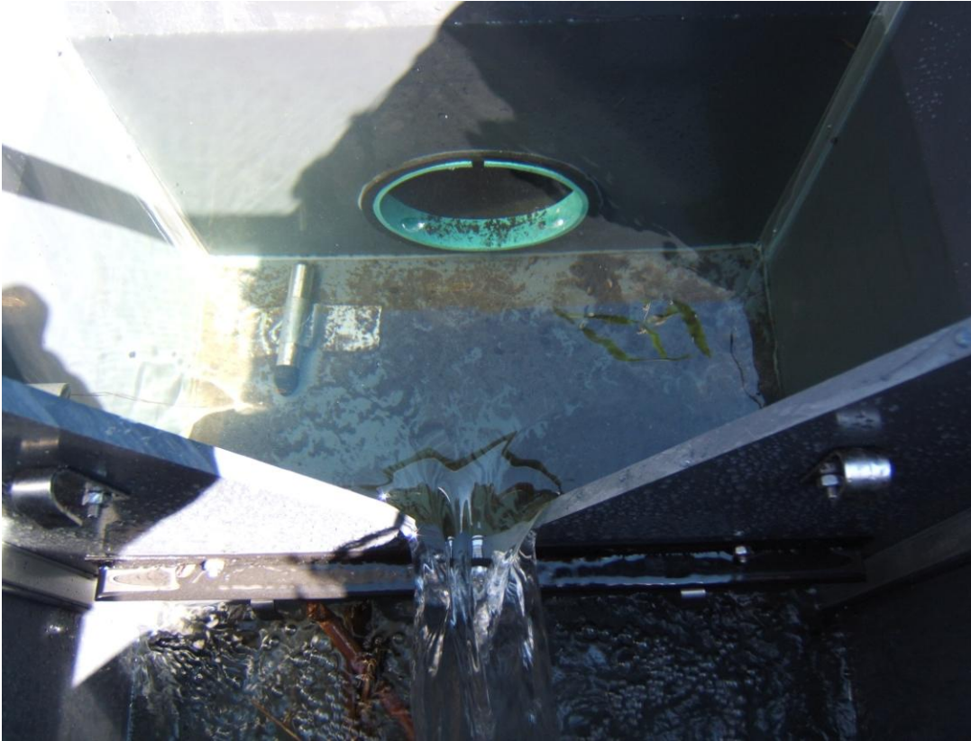
Figure 4. Water Control Structure for measuring flow from Bachand Tile Drainage
