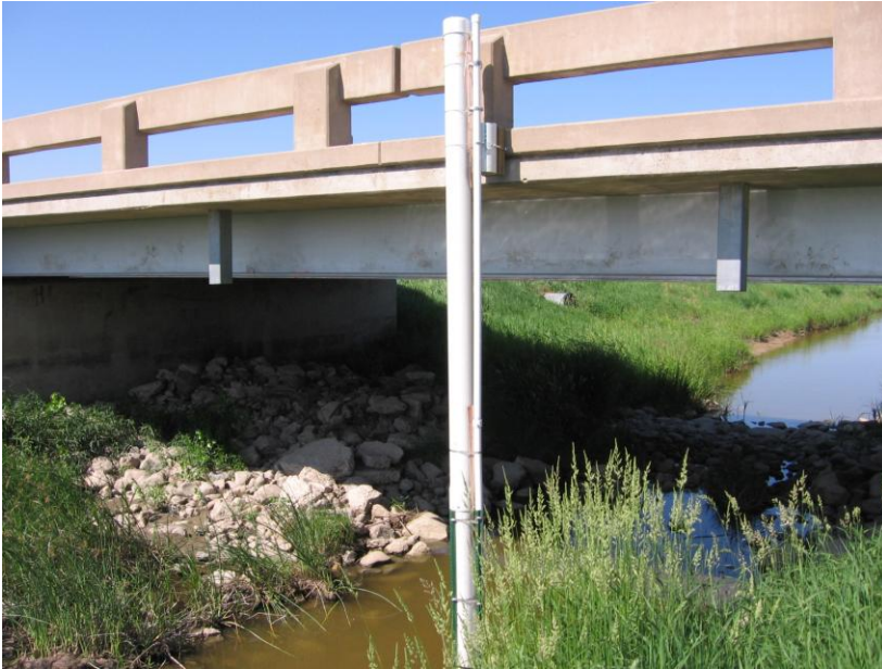
Figure 1. Stilling Wells for Turbidity and Water Level Sensors at Stream Gauge #71 on Polk County Ditch 2
