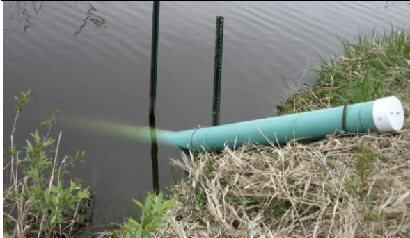
A4 (Ditch 200 entering Agassiz NWR) Water Quality & Level Logging Station
