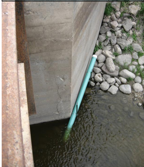
Stream Gauge 40 (Thief R./SD83) Water Level Logging Station
