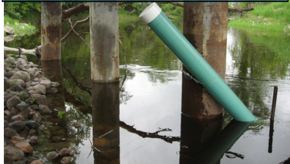
Site #760 (Thief R. at Hillyer Bridge) Water Level Logging Station
