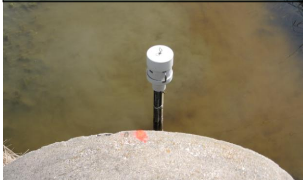
CD57 In-Situ TROLL 9000 Water Quality Logging Station
