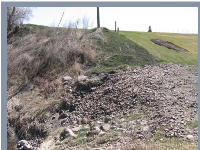
Erosion control by the Hill River in Brooks
