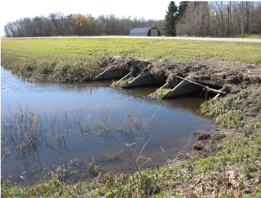
Debris piled on top of the culverts at the Hwy 54 crossing of the Moose River, indicating how high the water got in September.
